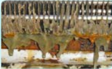
Mould inside refrigeration display
